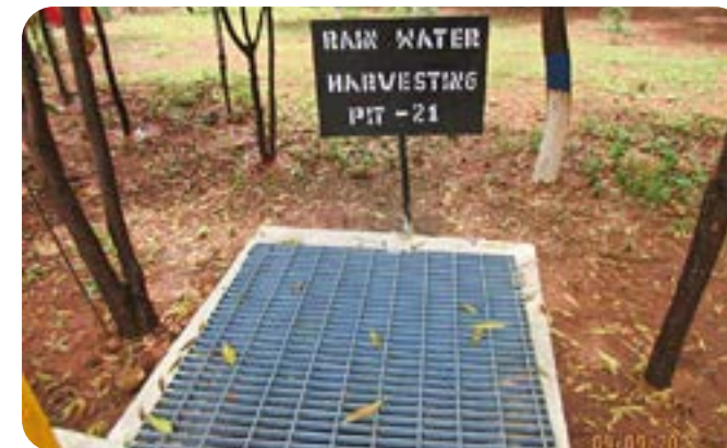
Rainwater Harvesting Pit
