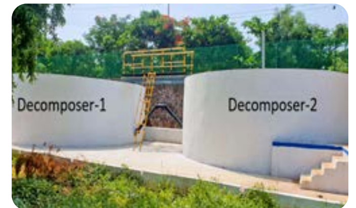
Biogas Preparation Facility
